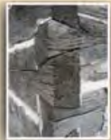
Dovetail corner joints have compound angles that naturally interlock the corner joints so they do not pull apart.
